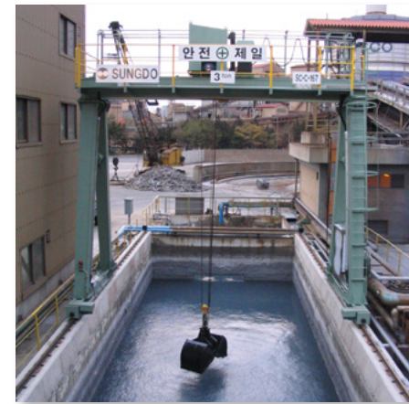
Bucket Hoist Crane
