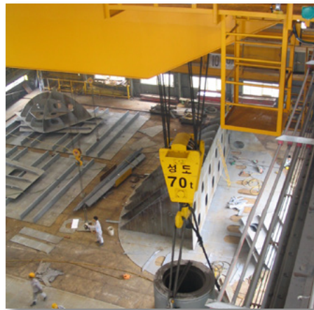
Double Overhead Hoist Crane
